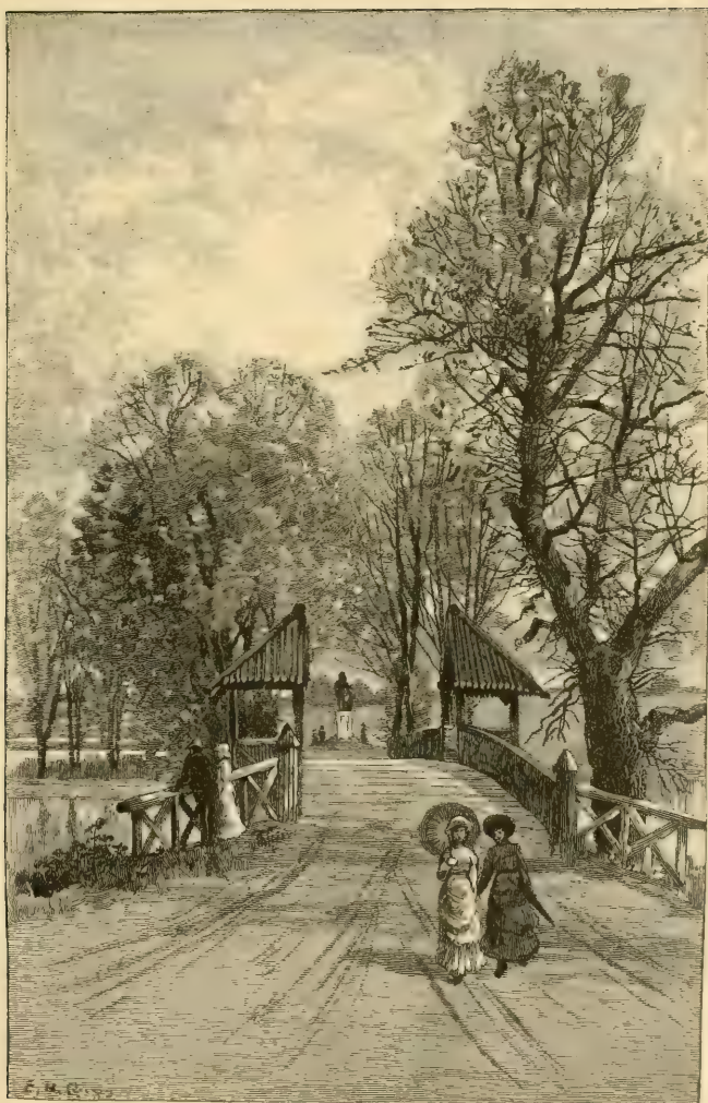
THE CONCORD BRIDGE.
